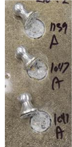
bulk concrete failures (ASTM D7234)
